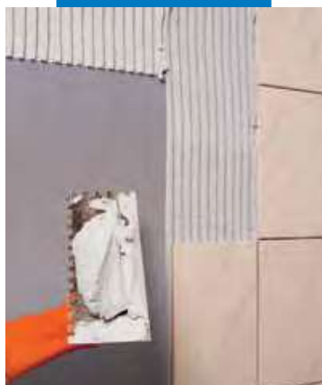
Mrázovka Tunnel - Prague - Czech Republic
