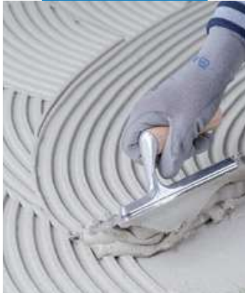
Spreading Adesilex P9 white
